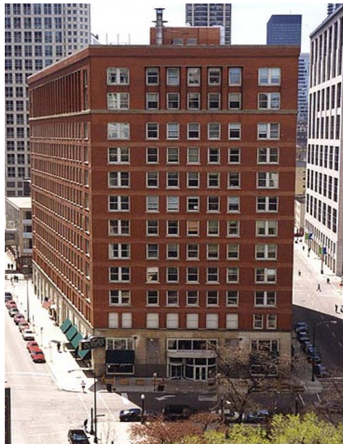
The RRB headquarters is located in the William O. Lipinski Federal Building, at 844 North Rush Street in Chicago, Illinois.
